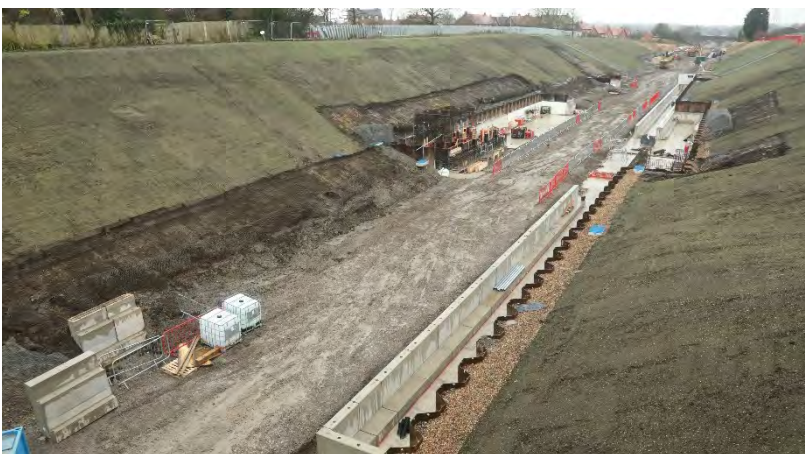
Winslow Station Platforms under construction in December 2021
