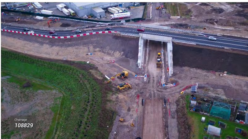
The second traffic switch for the construction of the new Charbridge Lane overbridge was completed in late 2021
